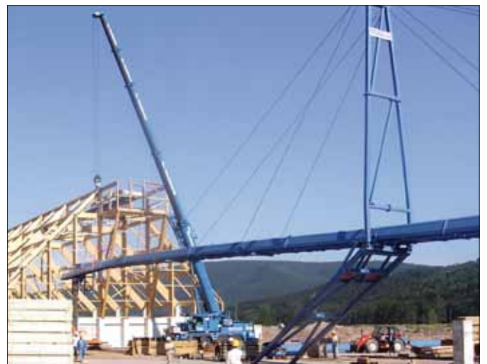
Lifting of pre-assembled sections
