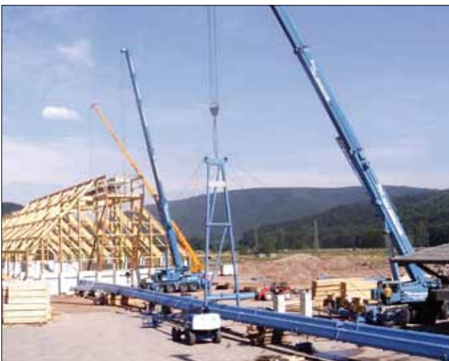
Assembly on the ground
